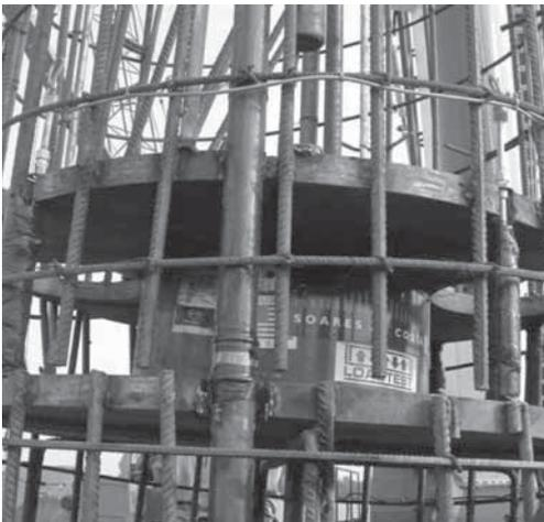
Figure 2. The reinforcing cage with the O-cell.
