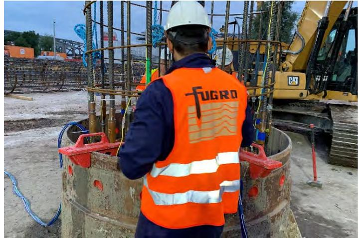
Pile reinforcement installation with O-cell® assembly
