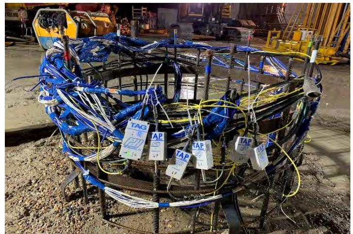
Thermal Integrity Profiling loggers
