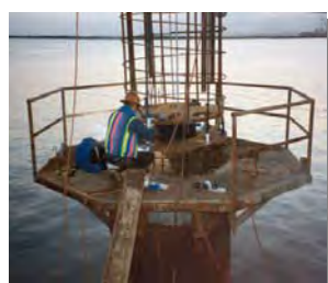
Installation of Pile Cage with O-cell assembly attached
