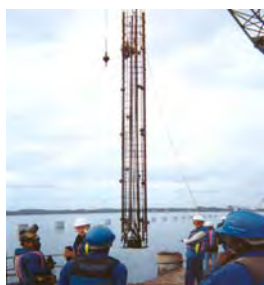
Pile cage showing O-cell assembly
