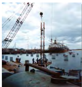
Pile construction offshore
