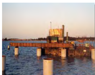
Pile test in progress
