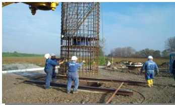
Installation of pile cage with O-cell assembly
