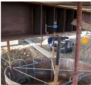
Pile test in progress
