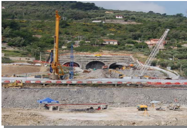
Testing of the 2000mm pile at Viadotto Imperia
