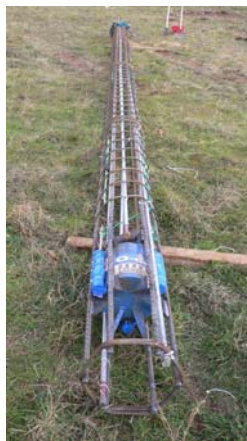
Reinforcing cage, O-cell and instrumentation ready for installation
