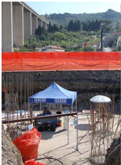
Testing of the 1400mm pile at Viadotto Prino
