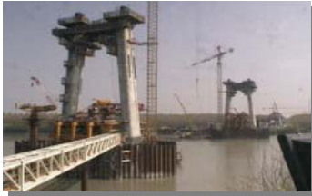
Construction of the bridge underway
