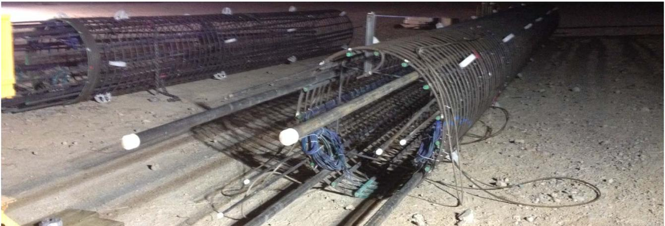
Shaft reinforcement with O-cell assembly.
