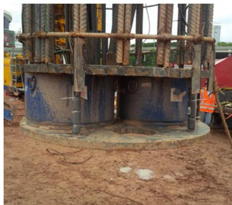
*O-Cell assembly at tip of reinforcing cage*
