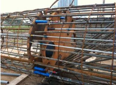
O-cell Assembly in Pile Cage (Bored Pile)
