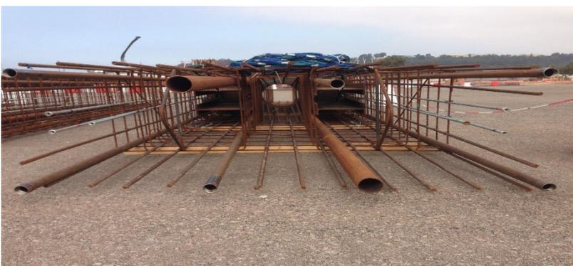
Full scale bi-directional static load testing using Osterberg-cells was utilised as the method which is specifically appropriate for the high test loads required on barrettes of this size and bearing capacity. The results obtained allowed confirmation, and potential optimisation, of the foundation design without the need for costly and time-consuming installation of reaction shafts used in traditional top down load testing.
