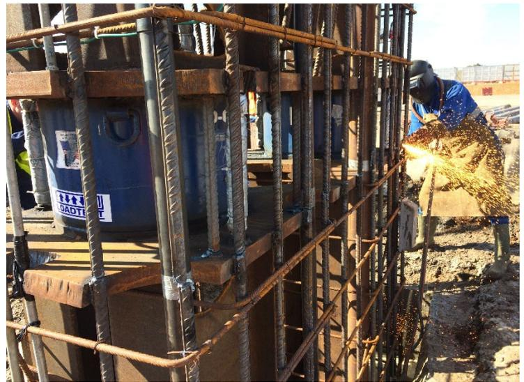
*O-cells positioned within their bearing plate assembly.
