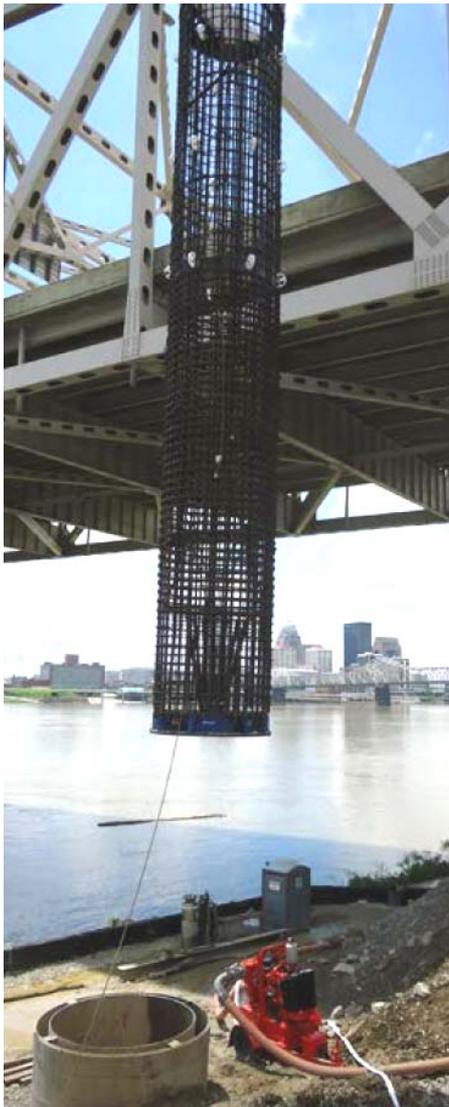
Reinforcement cage installation with O-cells
