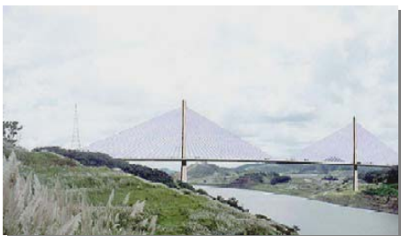
New Millennium Bridge over the Panama Canal Designers T. Y. Lin International Contractor: Bilfinger + Berger
