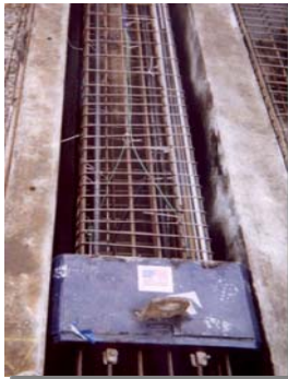
An O-cell assembly positioned in a 600mm square pile casting bed
