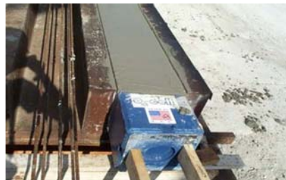
300x300mm O-cell concreted
