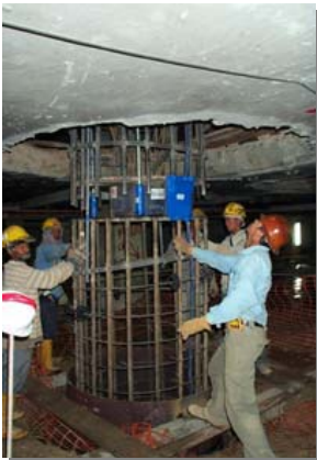
Installation through the basement levels
