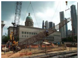
Placing cages within piles constructed in existing car park
