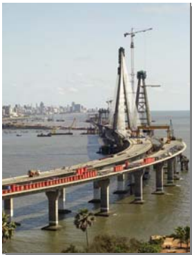
Under construction, May 2008
