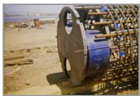
Lower level O-cell arrangement
