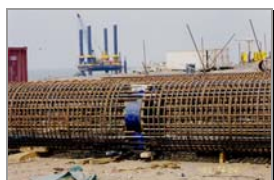
Upper level O-cell arrangement
