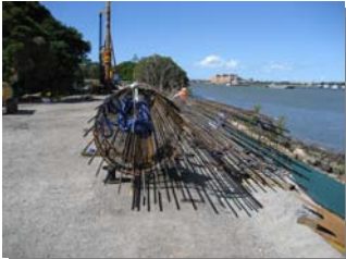
O-cell Cage ready for lifting
