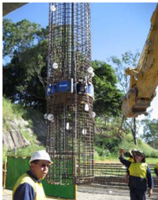
O-cell Assembly ready for placement
