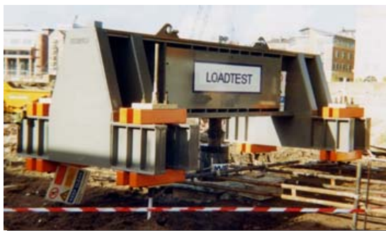
Figure 4. 4 MN CRAFT set up on 4 anchors with 4 Dywidag bars
