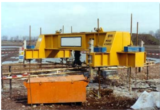
Figure 3. 2 MN CRAFT set up on 6 anchors with 6 Dywidag bars
