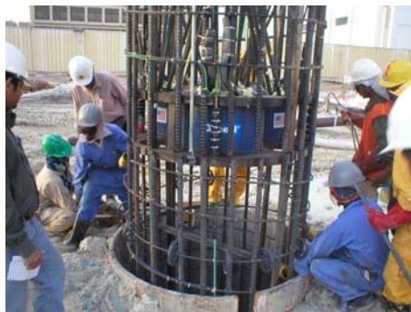
O-cell assembly being installed in Doha, State of Qatar
