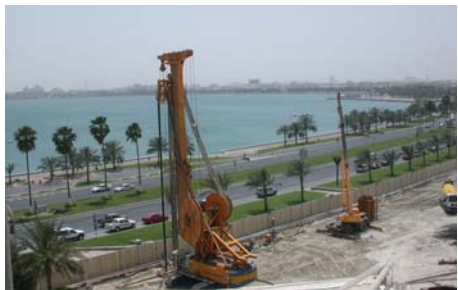
One of many projects along Al Corniche, Doha
