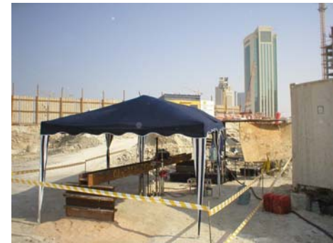
Load testing in progress
