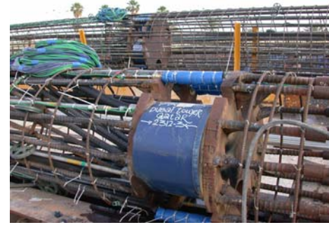
Several O-cell assemblies ready for installation.
