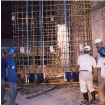
Installation of O-Cells into a slurry filled barrette
