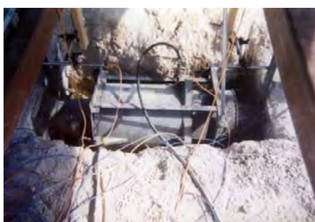
Conventional lateral load test
