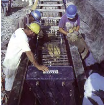
Installing an O-cell into a precast pile
