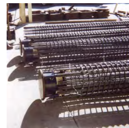
Testing multiple test piles
