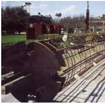
Single level O-cell assembly ready to install
