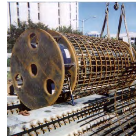
High capacity testing with multiple O-cells
