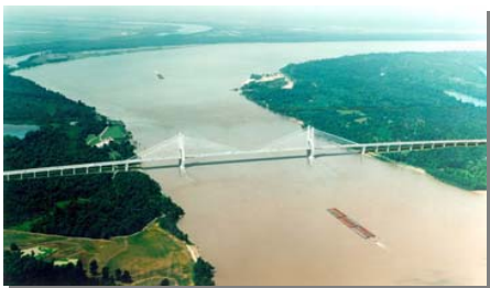
Hwy #82 Greenville Mississippi, USA Designers: HNTB Corp, Contractors: Massman Traylor Bros.
