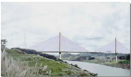
New Millennium Bridge over the Panama Canal Designers T. Y. Lin International Contractor: Bilfinger + Berger
