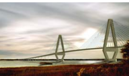
Cooper River Bridge in Charleston South Carolina Department of Transportation and Parsons Brinckerhoff, Trevlcos Corporation and Case Atlantic Co
