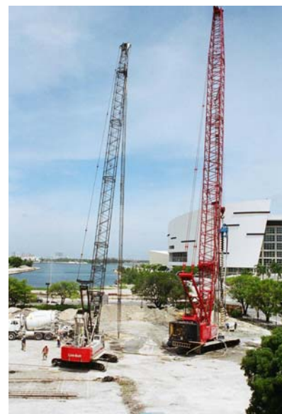
Cage & O-cell ready for installation
