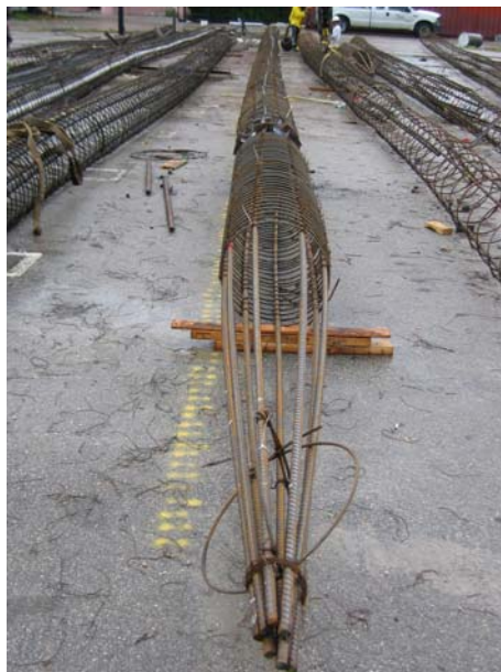
CFA/O-cell Assembly Tip
