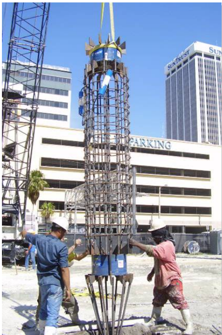
Assembly of a multi-level O-cell arrangement
