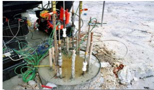
+20 MN CFA test in progress
