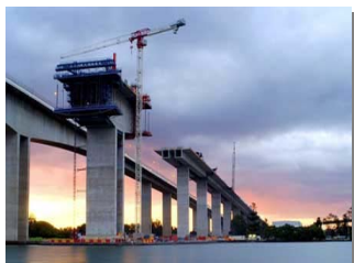
May 2009-Construction of the main span
