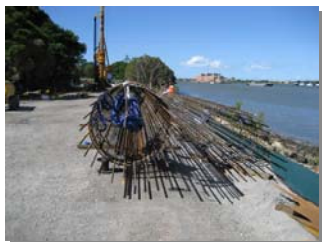
O-cell Assembly ready for placement
