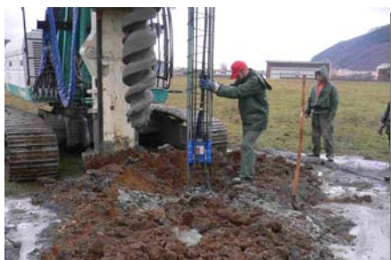
Installation of the single O-cell in a 450 mm pile
