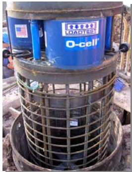
Installation of the lower assembly arrangement with 3x 405mm diameter O-cells
