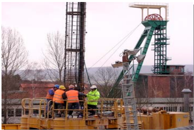
Installation of test pile cage
