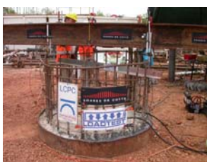
Bi-directional test in progress with steel reference beam for monitoring
