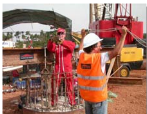
Installation of one of the removable extensometers
