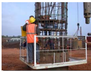
Installation of O-cell arrangement within pile cage
