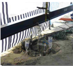
Pile head during testing
