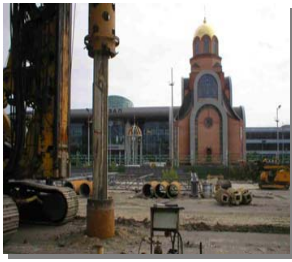
Piling opposite Voksal Central Train Station, Kiev
