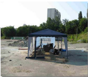
Pile test in progress protected from the elements
