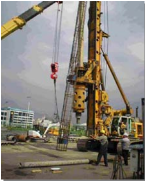
Lifting of multi-level cage at Solomenka, Kiev
