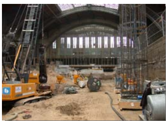
O-cell Assembly Placement
