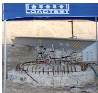
Pile head test arrangement showing reference beam
