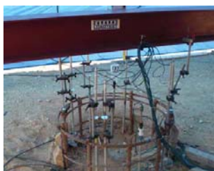
Testing in progress – pile head and reference beam
