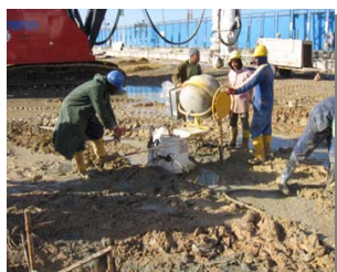
Post test grouting of a working pile
