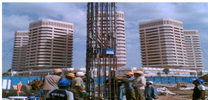
Installation of one of the preliminary test piles
