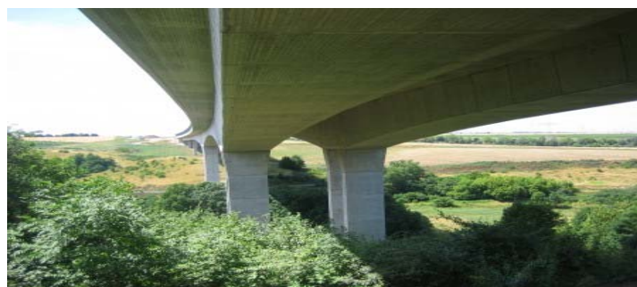
Underside of completed bridge
