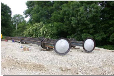
Installation of O-cells and pressure cell on the bottom of the carrying frame
