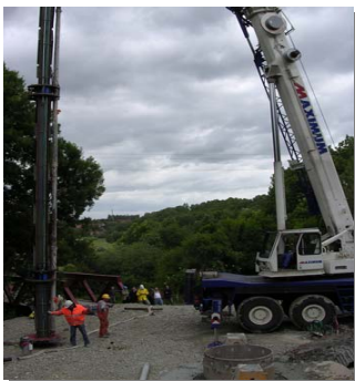
Lifting of the steel frame showing two O-cells at two levels
