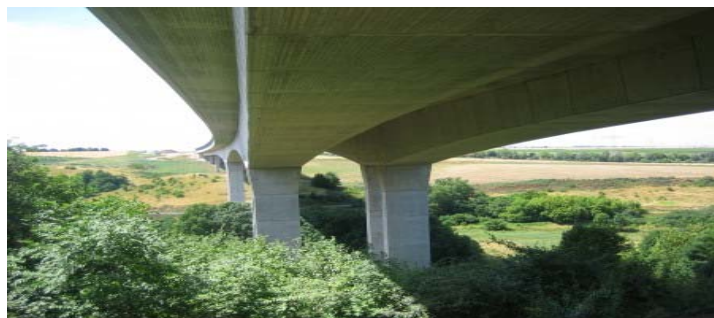
Underside of completed bridge
