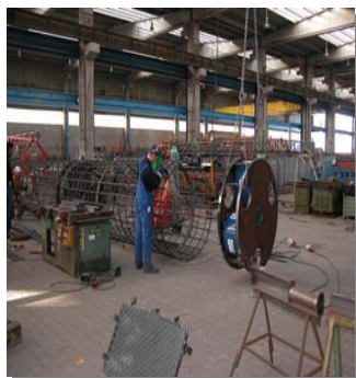
Cage assembly off-site
