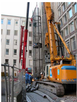
Installation of the bottom section of reinforcing cage
