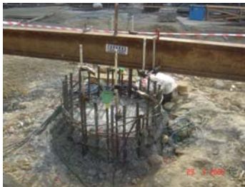
Pile Test Set-up Flame Towers
