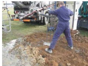
Installation of 'dummy' O-cell
