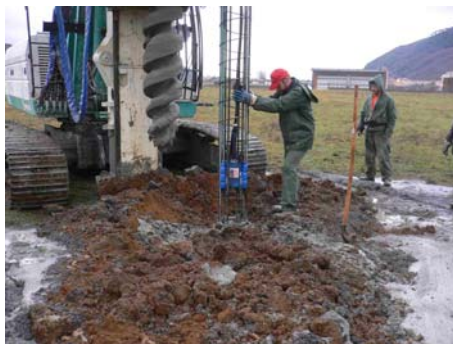
Install of the single O-cell in a 450mm pile
