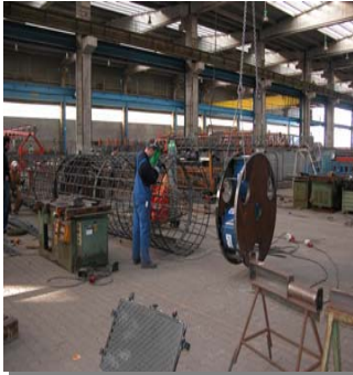
Cage and O-cell assembly fabricated off-site
