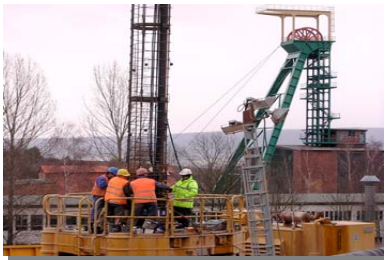
Installation of test pile cage
