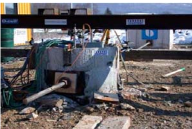
Lateral testing in progress
