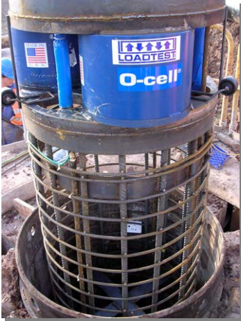
Installation of the lower assembly arrangement with 3x 405mm diameter O-cells
