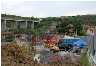
Testing of the 1400mm pile at Viadotto Caramagna
