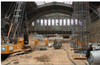
O-cell Assembly Placement
