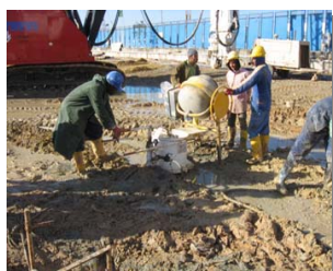
Post test grouting of a working pile
