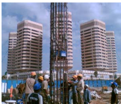
Installation of one of the preliminary test piles
