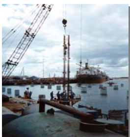
Pile construction offshore
