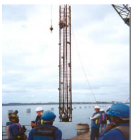
Pile cage showing O-cell assembly
