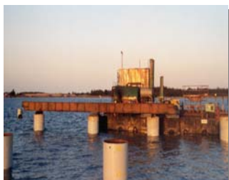
Pile test in progress
