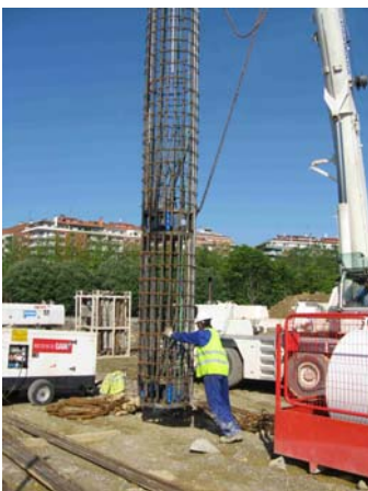
Multi-level cage layout before installation
