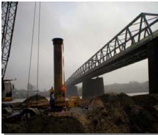
Test pile construction showing the previous bridge over the Rhine
