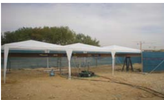
Bi-directional test in progress
