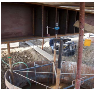
Pile test in progress
