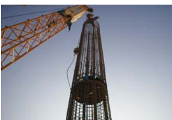
Installation of O-cell arrangement within pile cage
