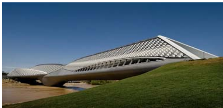
The Pavilion Bridge
