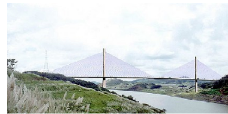
Second Bridge over the Panama Canal Designers T. Y. Lin International Contractor: Bilfinger + Berger
