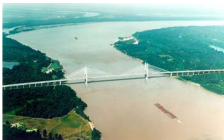
Hwy #82 Greenville Mississippi, USA Designers: HNTB Corp Contractors: Massman Traylor Bros.
