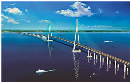
SuTong, China Design: China Highway Planning and Design Institute, Consultants Inc. (Beijing)
