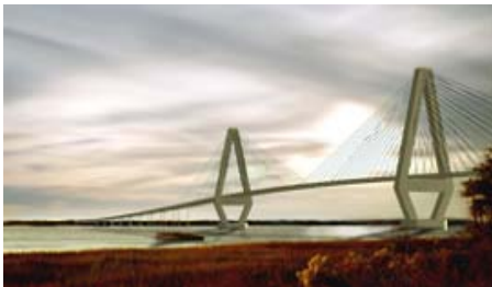
Cooper River Bridge in Charleston South Carolina Department of Transportation and Parsons Brinckerhoff, Trevlcos Corporation and Case Atlantic Co
