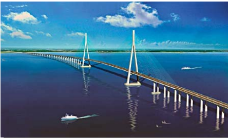
SuTong, China Design: China Highway Planning and Design Institute, Consultants Inc. (Beijing)
