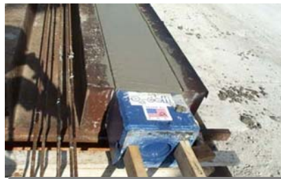
300x300mm O-cell concreted
