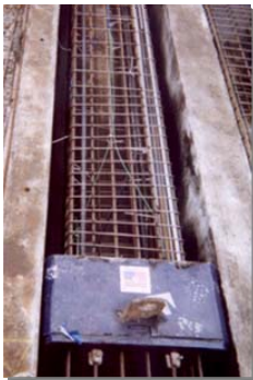
An O-cell assembly positioned in a 600 mm square pile casting bed
