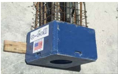
300x300mm O-cell before concreting
