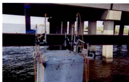
O-cell test on a 600 mm square pre-cast concrete pile being performed over water
