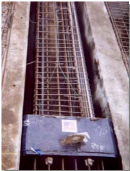
An O-cell assembly positioned in a 600mm square pile casting bed
