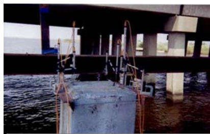
O-cell test on a 600 mm square pre-cast concrete pile being performed over water
