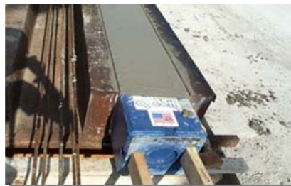
300x300mm O-cell concreted
