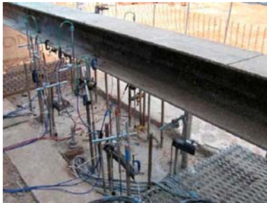
Test in progress: Instrumentation is installed throughout the barrette section and length
