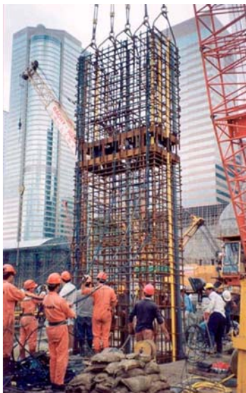
Cage Placement with O-Cells
