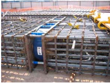
O-cells are installed within the barrette reinforcement
