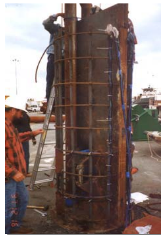
An O-cell® assembly is prepared for installation using two 4 MN (900 kip) cells for use in a 1200 mm (48") diameter shaft.
