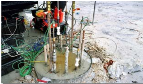
+2,000 Ton Augercast Test in progress
