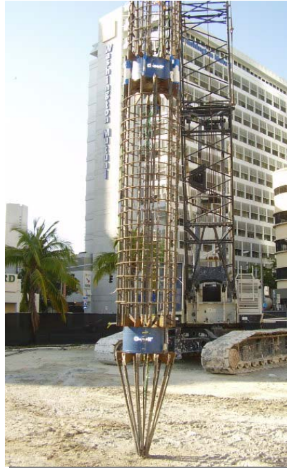
Assembly of a multi-level O-cell arrangement
